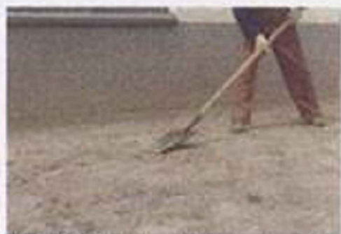
场地细平整，拍细，压实 (用碌筒子压实)
